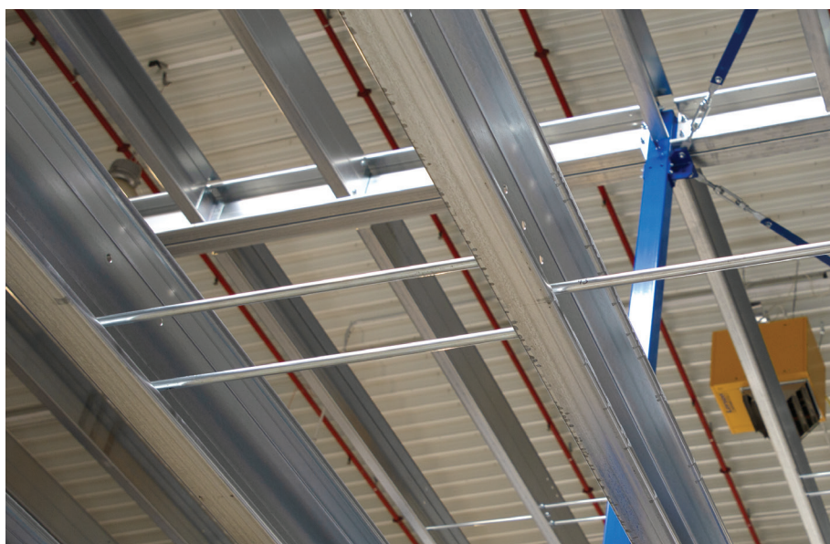
Fig. 25 – Diagram of the stiffening bars in a layout with an odd number of floor beams
