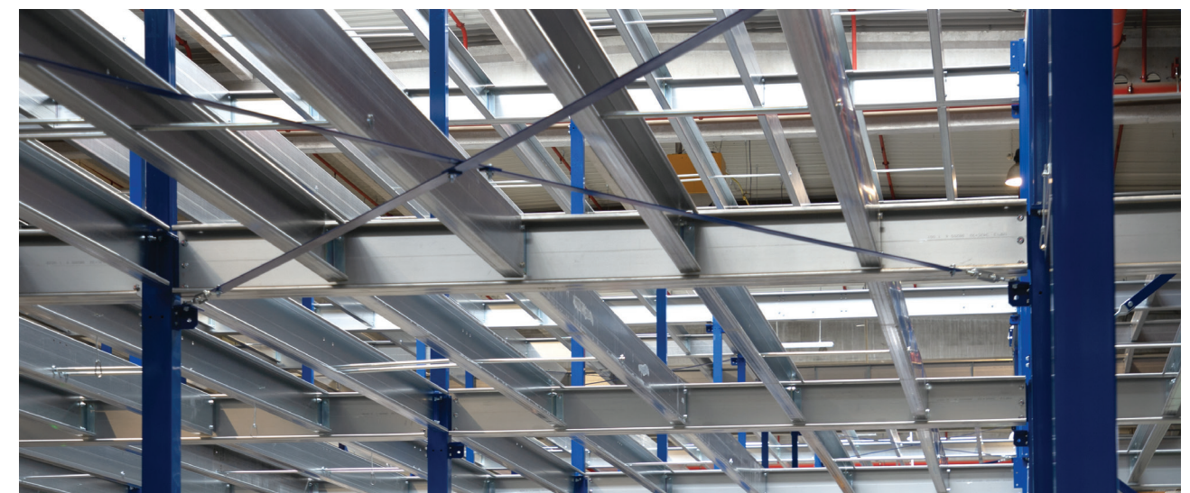
Fig. 13 – Girder connection to the column using one to three pairs of bolts
