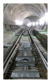
HYDROSTAR® is our complete solution in the field of innovative setting systems. In order to be able to meet your requirements in the high-performance range, we have developed a combined drive, locking and detection system for both switch assemblies and movable crossings. Ideal for use in high-performance tracks, the system features positive locking, even for the open switch blade. As an effective cost benefit for you, all variants only require one drive unit for integration into the signal box.
