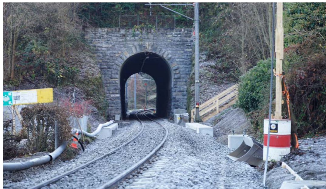
Construction site with typical sharp S-curve at Zentralbahn.
