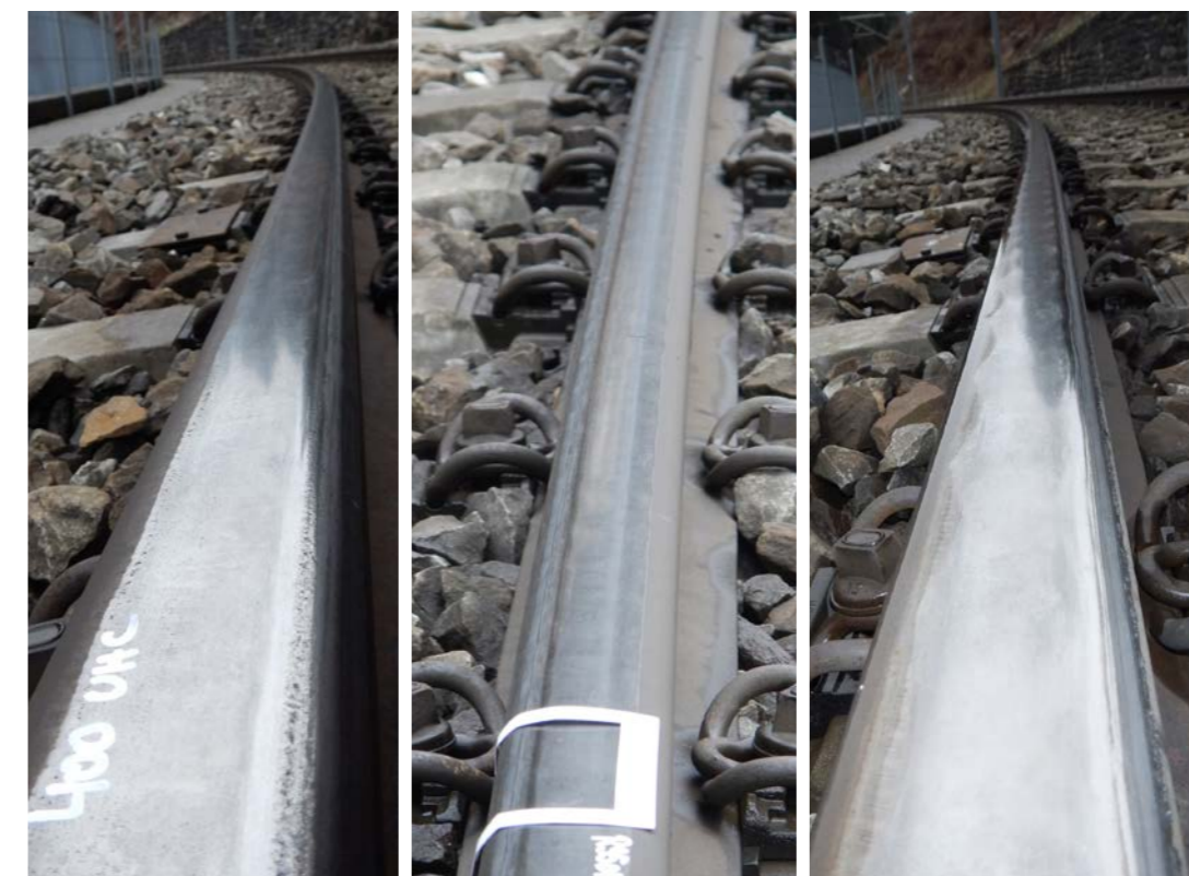
Corrugation of different rail types: (a) 400 UHC® HSH®, (b) R350HT and (c) R260 at RhB.
