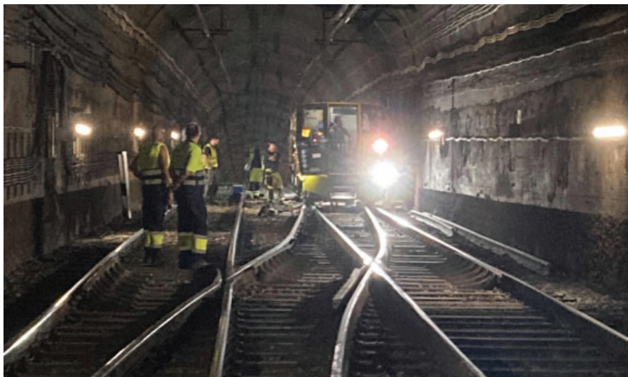
The MG11 machine can be fitted with special module to allow it to mill turnouts.
