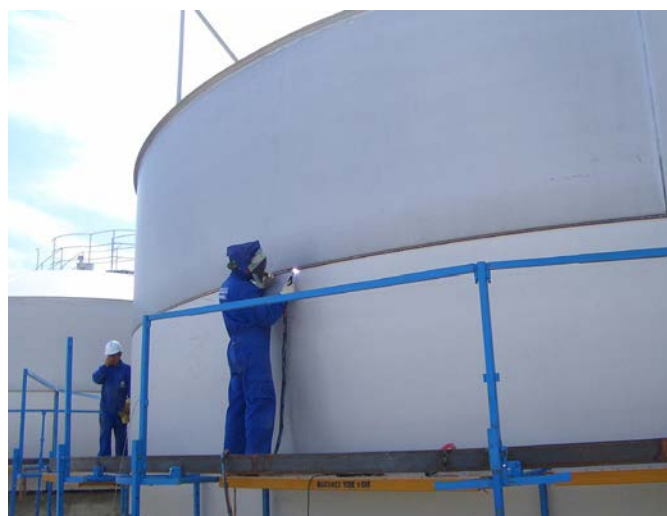
Welding on-site of stainless steel tanks – a typical application of Böhler Welding rutile all-position flux-cored wires. Tanks made of UNS S32101 and welded with FOXcore 2307-T1.
