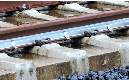
Route wiring with ClipFix
