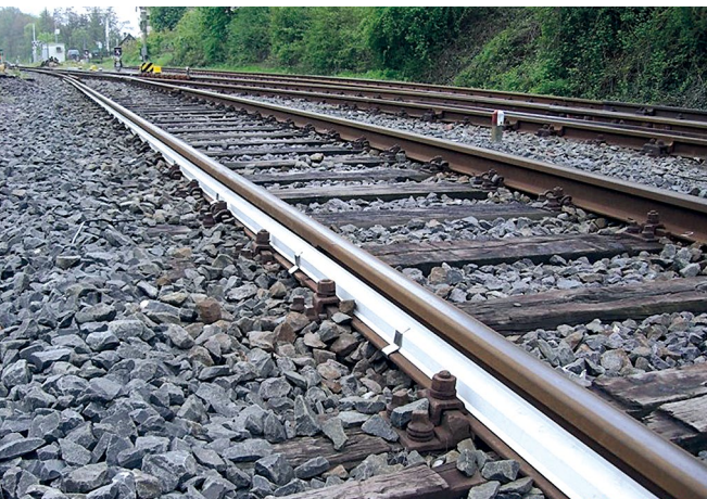
Route wiring with ClipFix
