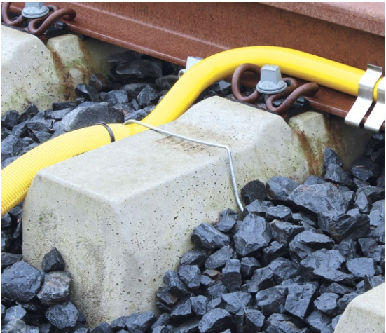
Fixation of the cable branch by means of sleeper clamps
