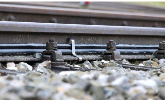
Rail foot clamp 2 mm with two cables
