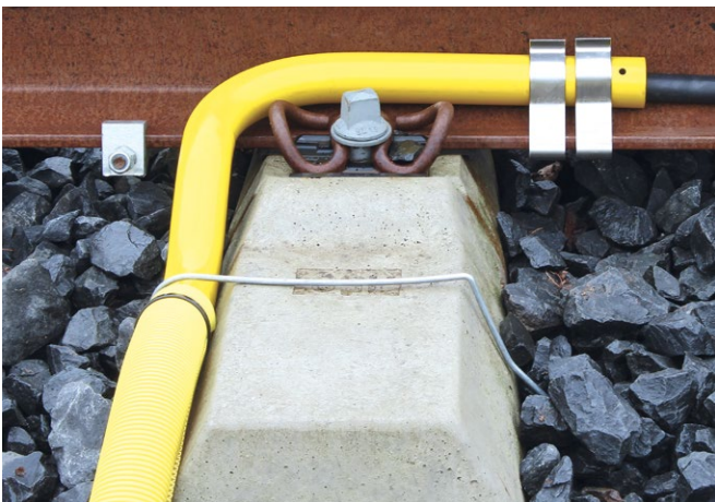
Fixation of the cable branch by means of sleeper clamps
