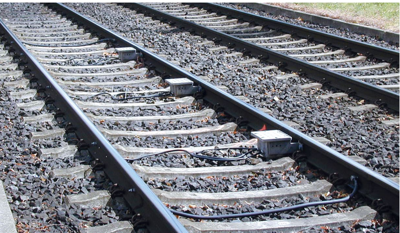
Lineside Boxes for track blocking circuit applications
