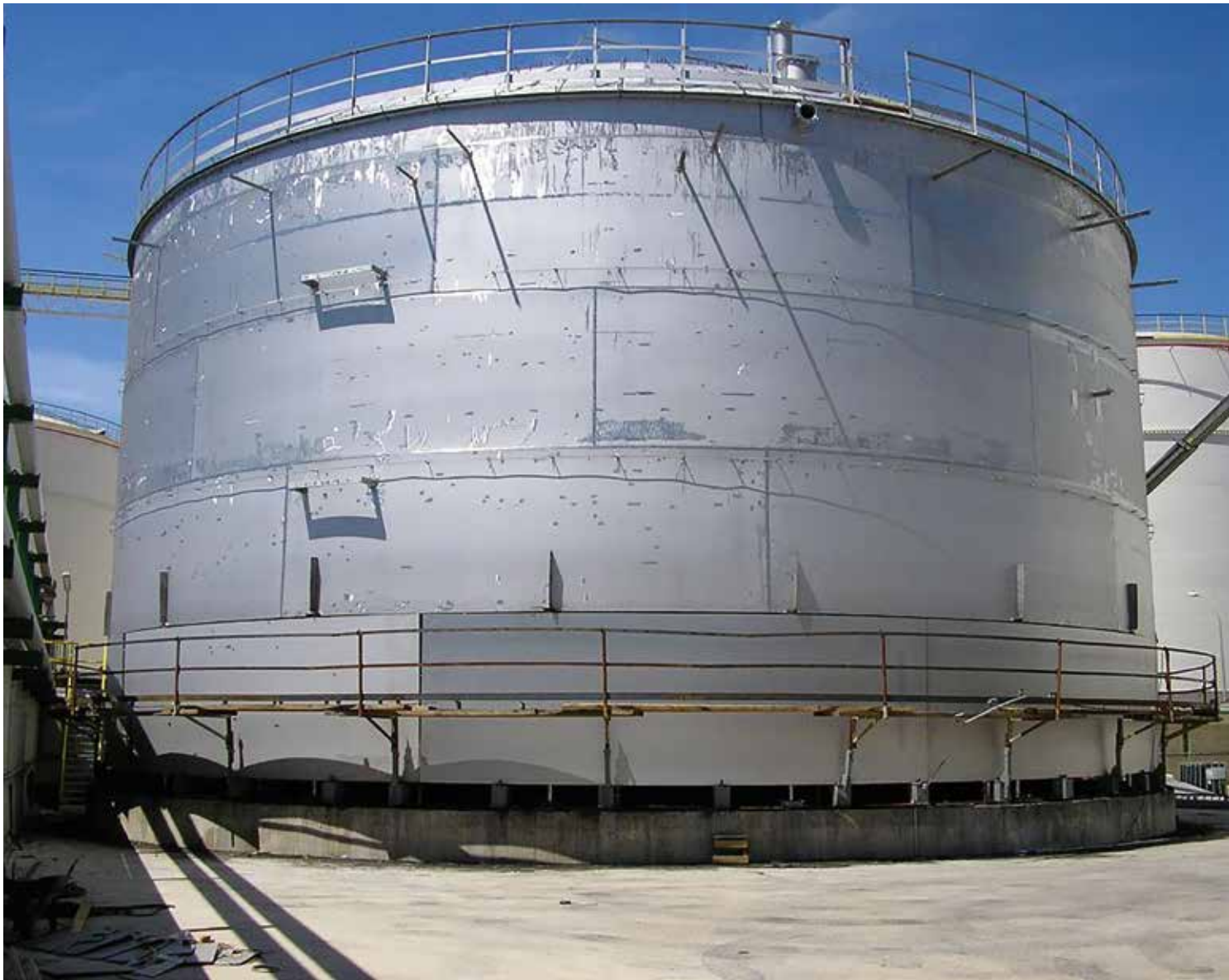
A pickled, duplex 2304 storage tank
