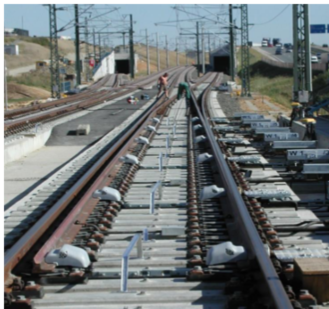
EW 60-10000/4000-1:39,173 fb with 6 HRS locking devices for sets of switches (NBS Köln-Rhein/Main, Breckenheim)
